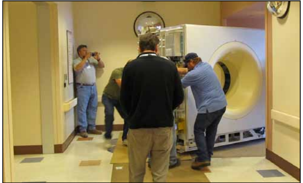
The 6,000-pound CT gantry is maneuvered down the hallway at NorthBay Medical Center last week.
