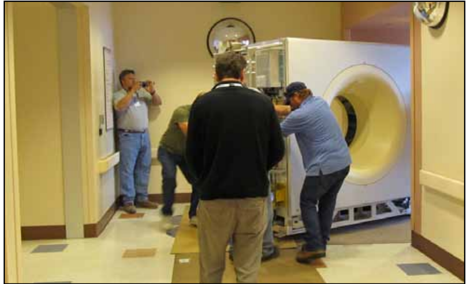
The 6,000-pound CT gantry is maneuvered down the hallway at NorthBay Medical Center last week.
